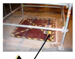
The warning sign here is a good example of additional marking on a protective cover.
