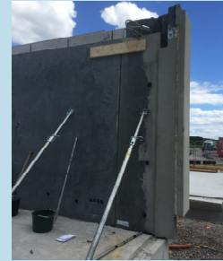
Wall support for prefab assembly
