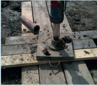
Load distribution for support legs
