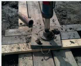
Load distribution for support legs.
