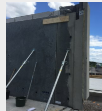
Wall support for prefab assembly .
